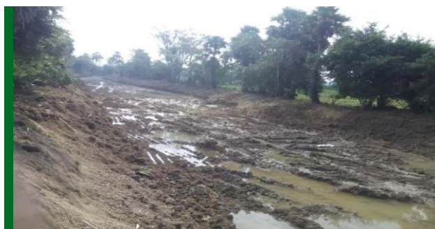
Channel after intervention
