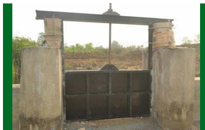
Check dam with percolation pond
