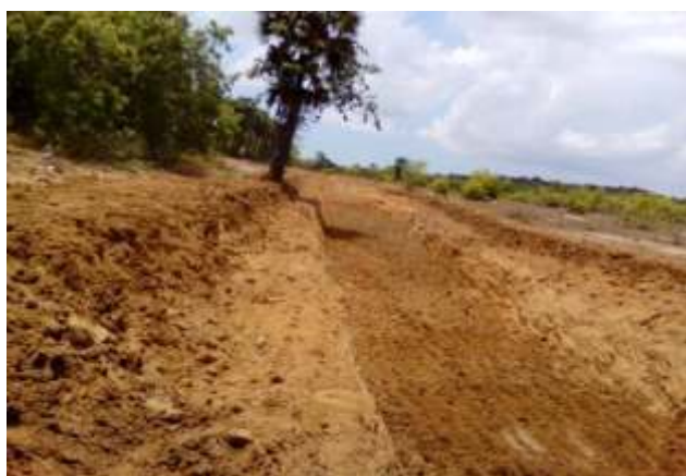
Photo: The channel is made for water drainage
