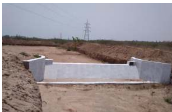
Photo: Check dam cum percolation tank
