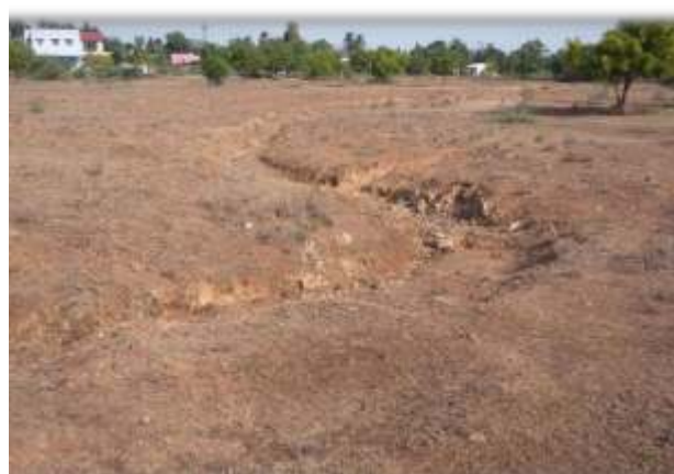
Photo: The channel is cleared for water drainage
