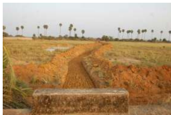
Photo: Construction of a channel to manage the flood
