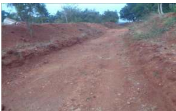
Photo: Channel cleared
