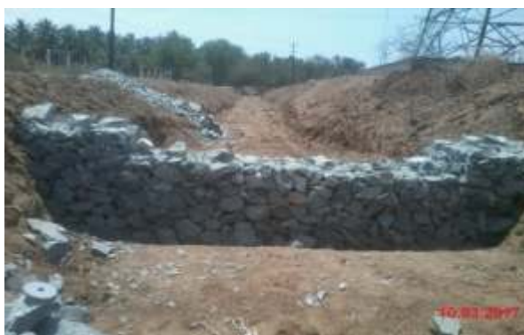
Photo: Gabion Check Dam
