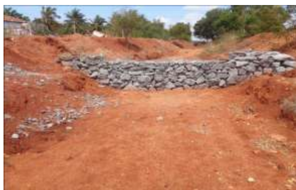
Photo: Gabion check Dam
