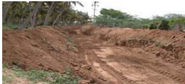
Photo: Channel after excavation
