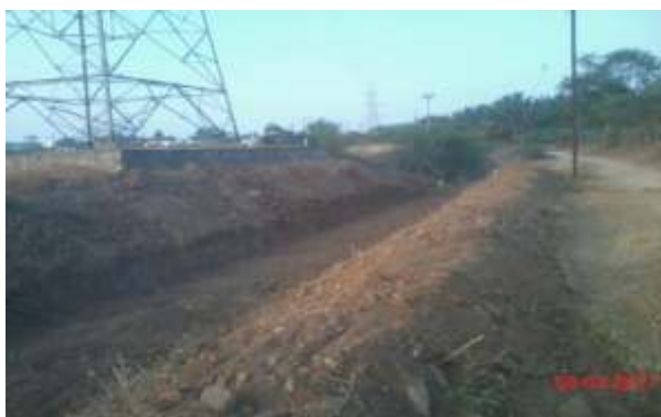
Photo: Channel cleared
