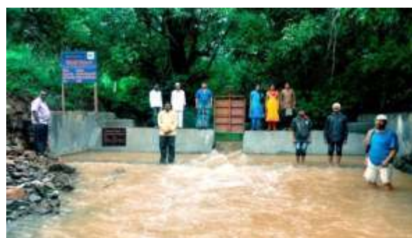
Project site after construction of farm pond at Kolvadi watershed, Pune
